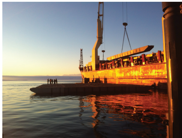
Figure 9-5. The Army’s 331st Transportation Company built the steel pier (pictured) when the ice pier used at McMurdo Station, Antarctica, failed. Supplies from the USNS Green Wave are being received on this pier.
